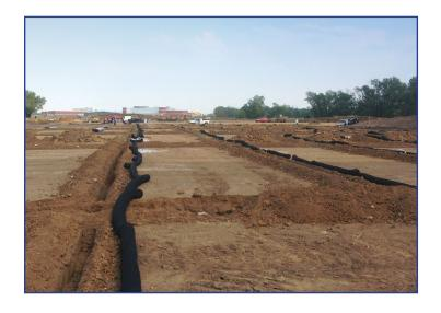
trenches filled with gravel, pipe and fabric. However, the contractor suggested an easier, better performing and more cost-effective drainage solution: **EZflow by NDS**.
