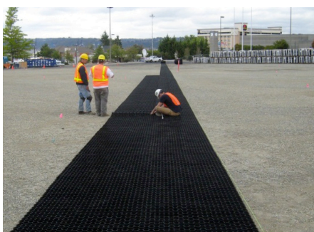
Installing EZ Roll after preparing and compacting sub-grade.
