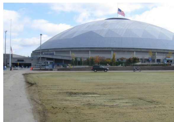
LeMay’s new automotive display area immediately following EZ Roll installation and hydroseeding.
