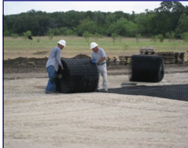
EZ Roll at the installation site; each roll is 600 sq ft.
