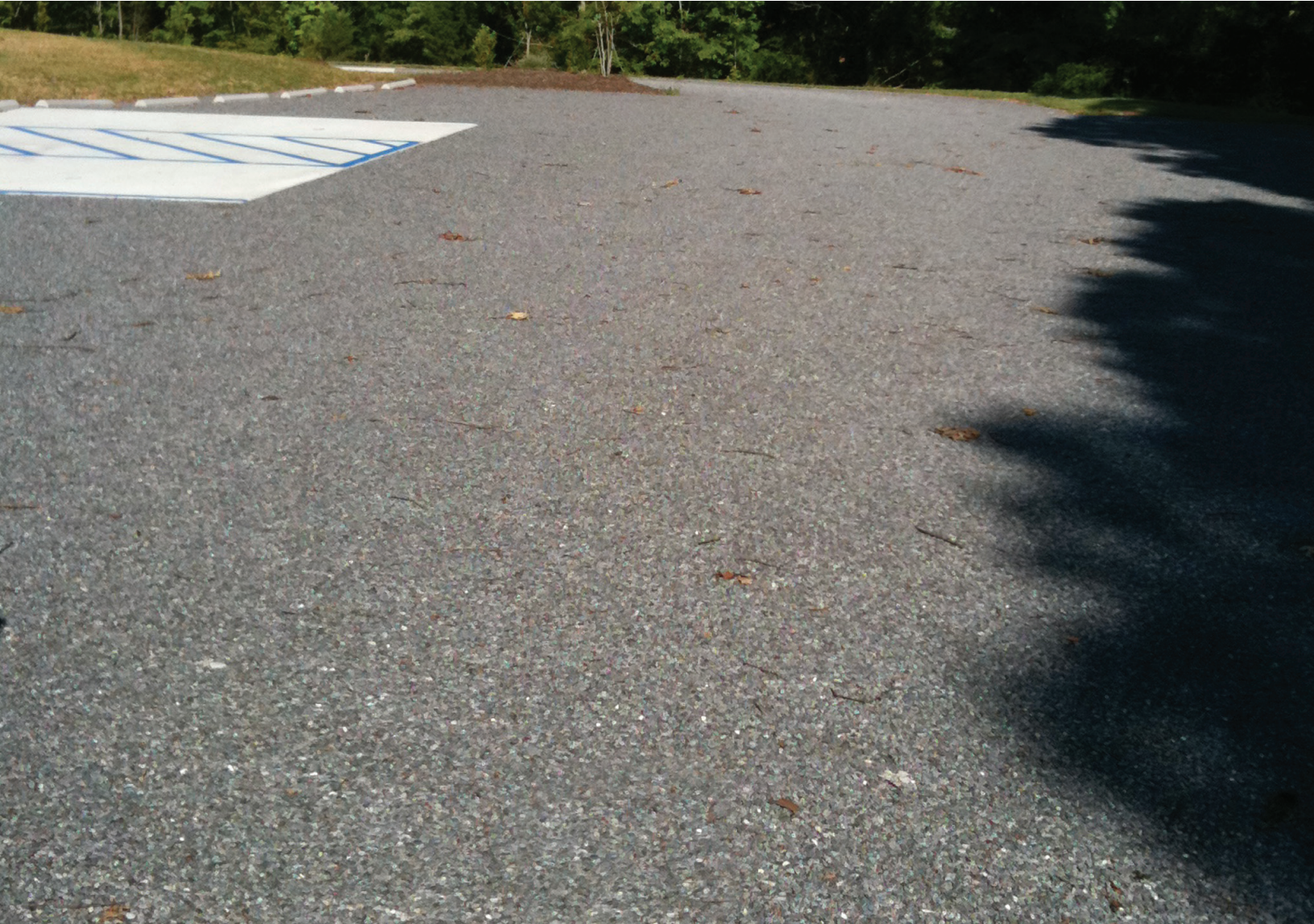
Above Right: Installed Paver. Above: Installation 1 year later, taken July 2011.
