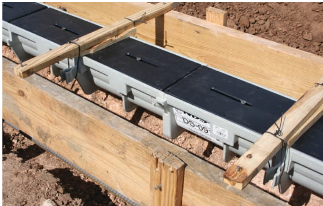
Dura Slope Trench Drain in section
