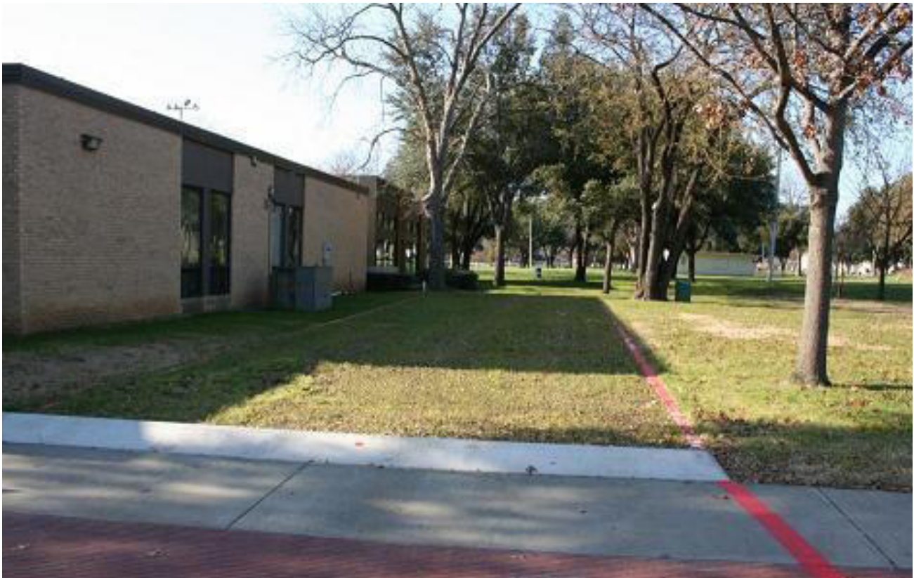
NDS EZ Roll Grass Paver was installed on the far side of the building to provide access for emergency vehicles.
