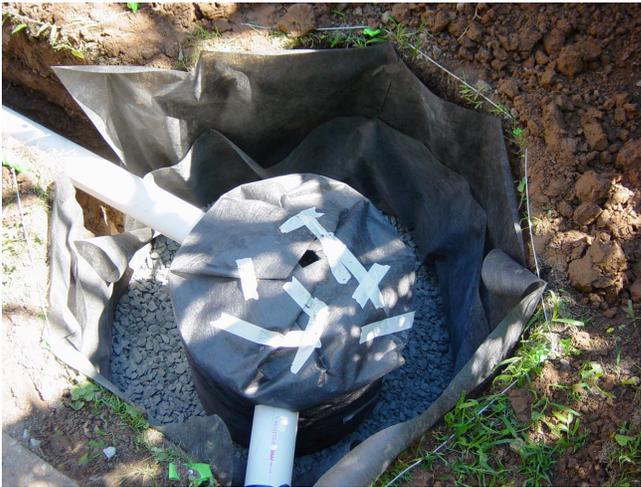
A four (4) foot deep by four (4) foot diameter hole was dug by hand to prepare for the Flo-Well. Geotextile was installed around the soil walls. One (1) foot of clean stone, sized    inch was placed on the bottom of the hole. The Flo-Well (wrapped in geotextile) was set and the drainage pipes were connected to the device. Stone was backfilled up to the top of the Flo-Well. Geotextile was placed on the top of the stone to permit the placement of eight (8) inches of soil to match original grade.
