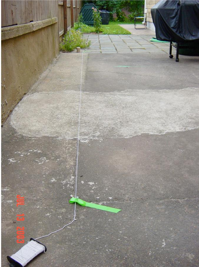
Two (2) separate conditions are believed to exacerbate the flooding of the basement. The first is a concrete low area that fills with stormwater runoff from a neighbor's roof. This area continues to be ponded until water seeps through expansion joints with help from evaporation.
