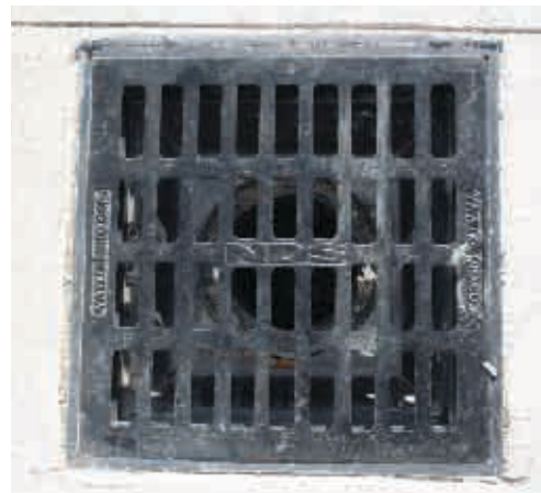
The NDS 18" square grate in cast iron
