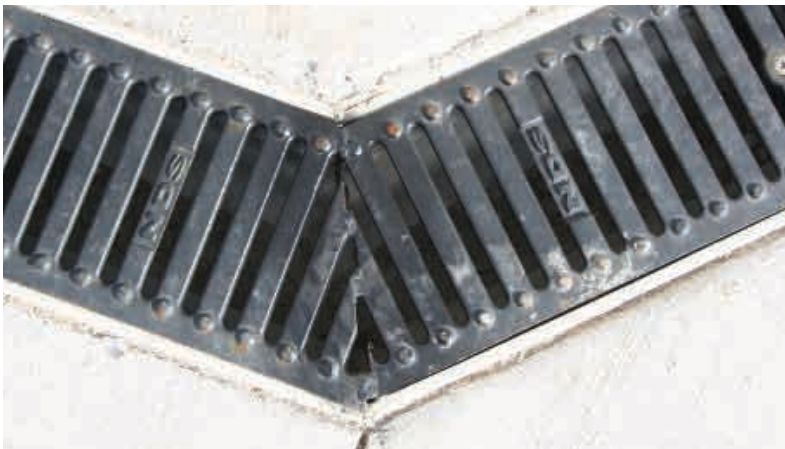
DS-231 cast iron grates were mitered and spot-welded to accommodate the custom angle above
