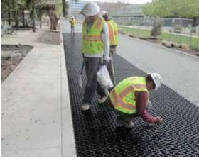
Here the contractor quickly assembles two lengths of EZ Roll Permeable Pavers. Using the integrated clips, assembling EZ Roll pavers sideto-side or end-to-end is easily accomplished without special tools.
