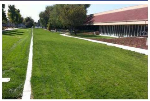
EZ Roll Permeable Grass Paver provides a lush green emergency access lane that blends into the landscape, reduces the amount of stormwater that enters the municipal system and filters pollutants typically contained in hardscape runoff.
