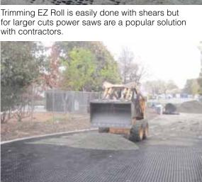
The empty compressive strength of EZ Roll readily supports the weight of equipment used to spread fill material. Fully loaded dump trucks can back onto EZ Roll to dump the material just where you need it.
