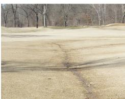
people on the job to trench and install the product that ended up taking 1 day to trench and install; 2 days to clean up spoils. If I had used pea gravel and pipe, I would have needed 7 guys for 7 days to trench, install and clean the site of excess gravel.
