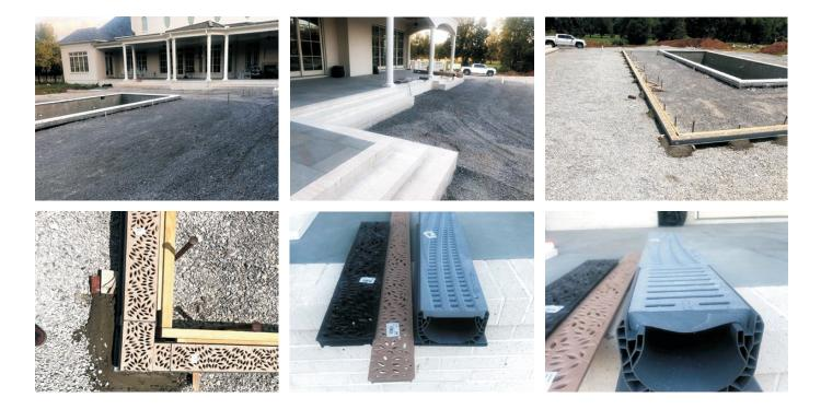
Combining a compact, reinforced channel and terrific grate options that support light vehicle loads, the SpeeD Channel is ideal for commercial and residential applications alike. The SpeeD Channel offers a variety of optional accessories that maximize water flow efficiency. At the end of the project, two separate 50' runs were installed around the exterior of the pool amounting to a total of 100 sq feet of SpeeD Channel.
