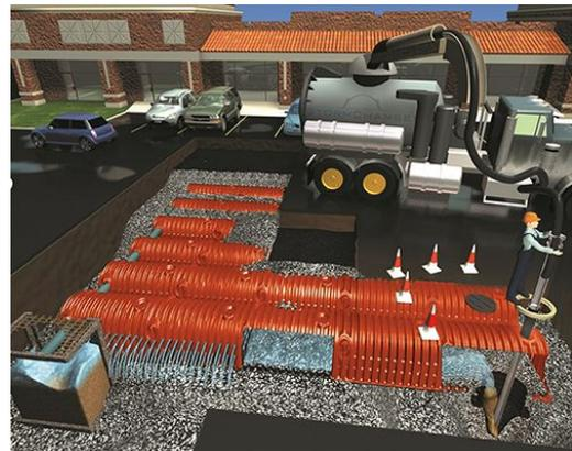
It is highly recommended that the StormChamber system not be opened to receive storm water flows until construction of the site has been completed. Even then, all storm water inlets must be protected from sediment loading until the site is completely stabilized. Complete stabilization implies that the construction site has been cleared of construction-related debris and has incurred at least two storm events sufficient to wash most soil and other particulate matter off impervious surfaces.
