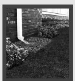
Catch basins and grates remove water from downspouts to protect your home's foundation and basement walls.
