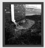
Excess water around the home cracks and damages the foundation and basement walls.
