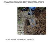
Dig holes and trench for pipe, Flo-Well, and EZ-Drain. Dry fit (no glue) the entiredrainage system from the Flo-Well to the pop-up emitter. The Flo-Well and EZ-Drain should be installed at least 10' away from any existing structure. Measure and cut all pipe to necessary lengths. After completing each step, glue parts together.
